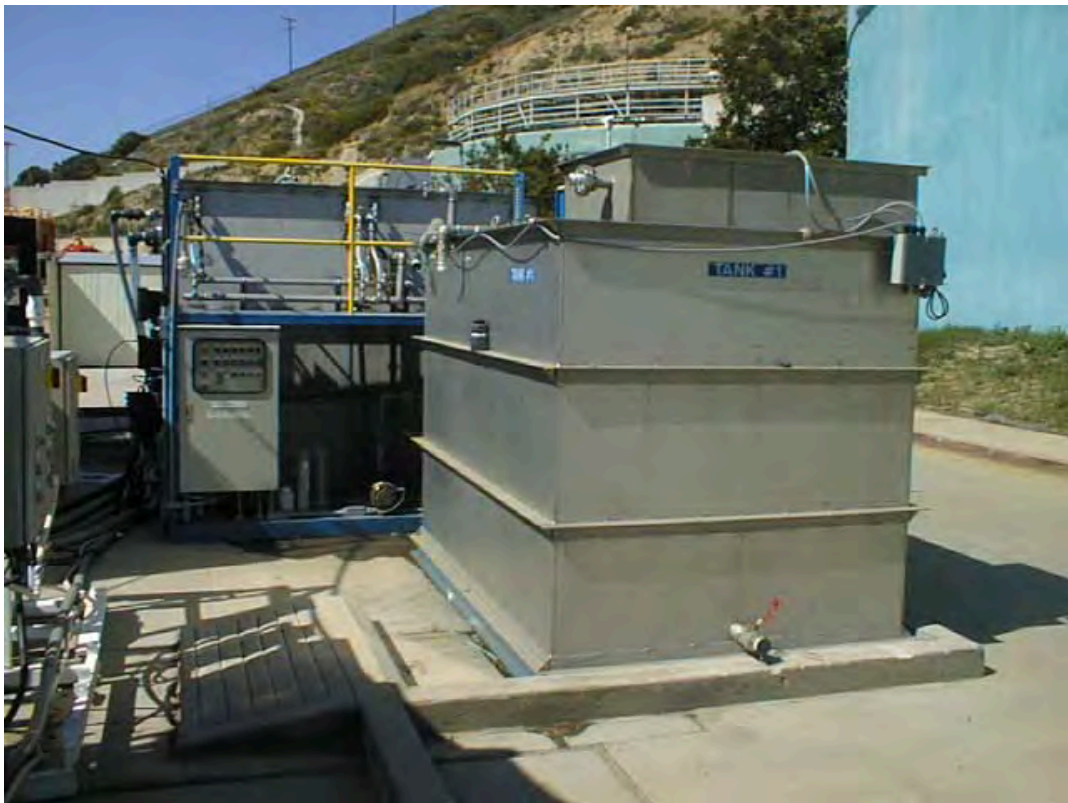
Mitsubishi MBR Pilot Unit (front view)
