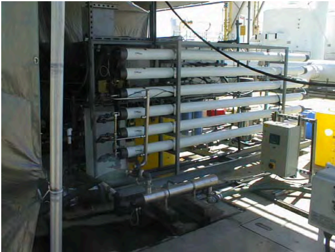
RO Pilot Skid
